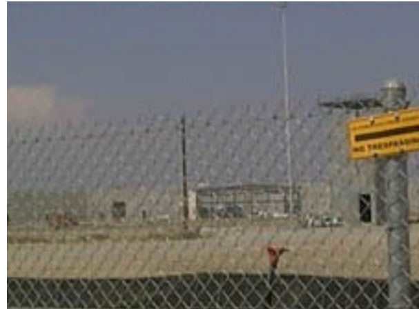
Delano II Prison Under Construction
